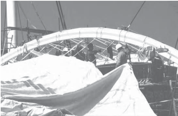
12.7 Stressing out the membrane at the Inland Revenue amenity building, Nottingham (photo: Alistair Gardner).
