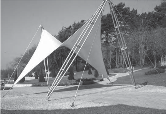
12.1 Simple anticlastic form of a small canopy, Millennium Garden, University of Nottingham, UK. The form has two high and two low points creating a classic saddle surface (photo: John Chilton).
