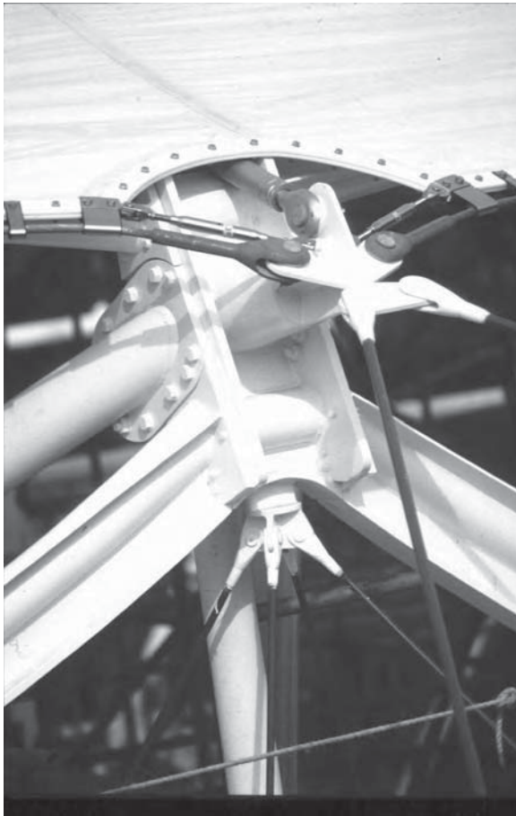
12.8 Cable and edge details, Inland Revenue amenity building, Nottingham (photo: Alistair Gardner).
