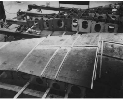
Steel Plates and Eggcrate Substructure
