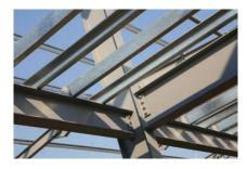
Beam-to-column connection with one beam attached to column flange and other attached to column web
