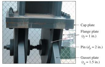
(b) Detail at bottom of brace
