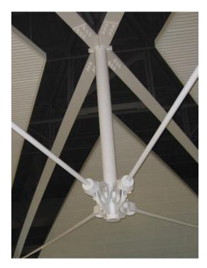
Cable and strut at typical joint of airport concourse roof
