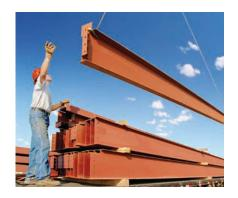
Bending due to self weight of beam and axial compression due to horizontal component of cable lifting force
