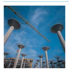
Slender concrete columns fixed at the base and free at the top during construction
