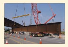
Bridge girder with overhang during transport to the construction site
