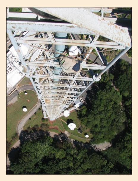
This telecommunications tower is an assemblage of many members that act primarily in tension or compression.
