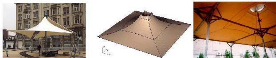
Fig. 9. (a) Tolerant tensile border saddle configuration. (b,c) Sensitive Mina valley tent
