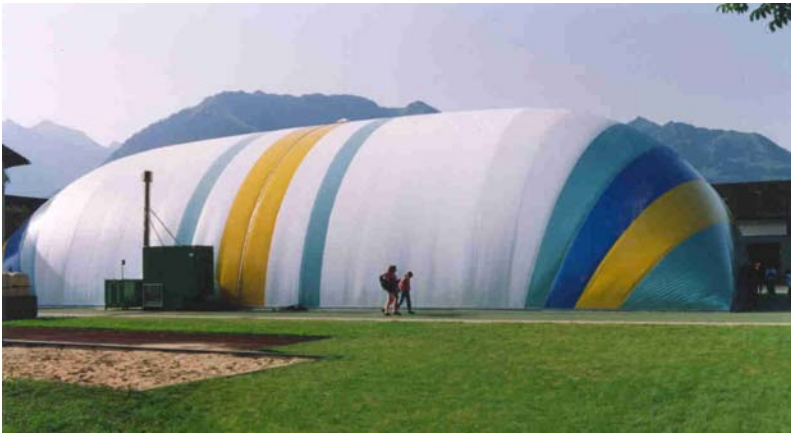
Fig. 6. Tennis court cover [6], permanent
