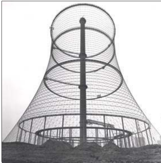
Fig. 2. Cooling tower Schmehausen [2], permanent
