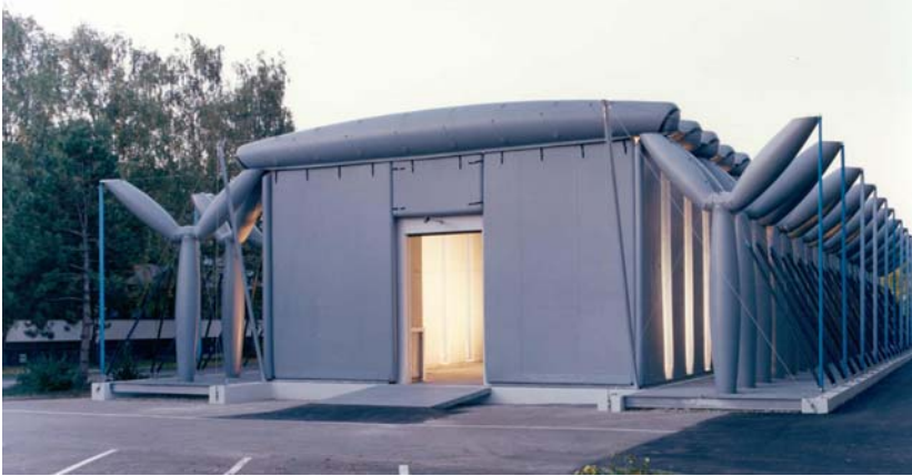
Fig. 3. Festo-building in Stuttgart [3], permanent
