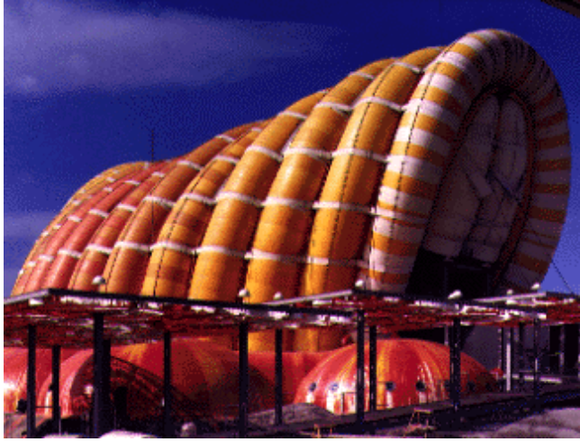
Fig. 1. Example of inflated pavilion formed by assembly of high pressure tubes. “Fuji” Inflatable pavilion constructed by Mamoru Kawaguchi in 1974 for the “Expo Tokyo”
