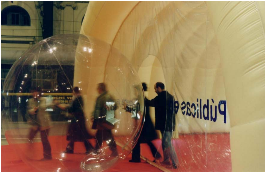
Fig. 18. Door detail, formed by an inflatable ball
