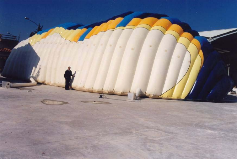
Fig. 4. Inflatable pavilion ( 250\text{m}^2 ) formed by an assembly of low pressure tubes built for the mobile exhibition for the Gaudi Year of Construction Artisans, Barcelona 2002
