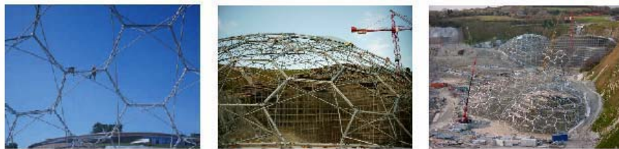
Figs. 39-40. Eden Project, Cornwall, GB, Nicholas Grimshaw Architects, Anthony Hunt Associates engineers, structure: MERO Membrane ETFE-Pillows diameter 9 m, Dimensions: 15 590m 2 , 100m × 220 m height 55 [www.anthonyhuntassociates.co.uk]
