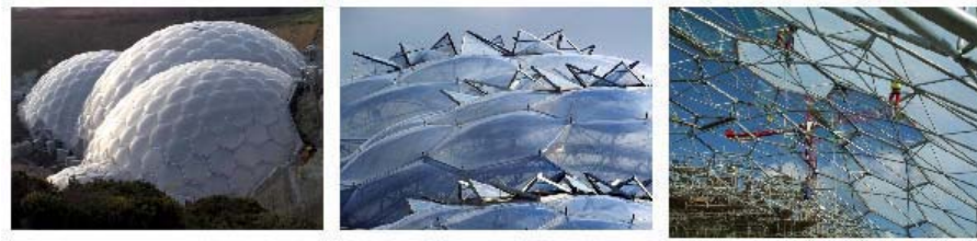
Figs. 41-43. The transparent foil 'windows', made of 3 layers of ETFE (ethylenetetrafluoroethylene-copolymer), form inflated 2- metre-deep pillows. ETFE has a lifespan of over 25 years, transmits UV light, is non-stick, self-cleaning and weighs less than 1/10th the equivalent area of glass and has a great stress redundancy. [www.anthonyhuntassociates.co.uk]
