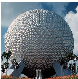
Fig. 36. Geodesic sphere
